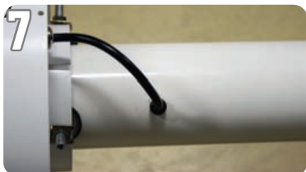
7 Press the grommet tightly into the pole to prevent moisture
