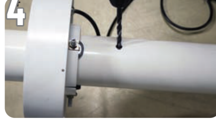
4 Drill a 3/8" hole beneath unit for cable access
