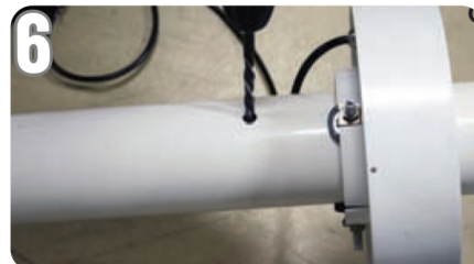
6 Pull cable through the pole*
