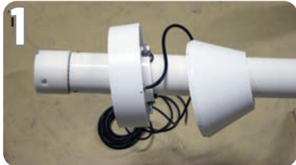
1 Slide cover and light unit onto the pole
